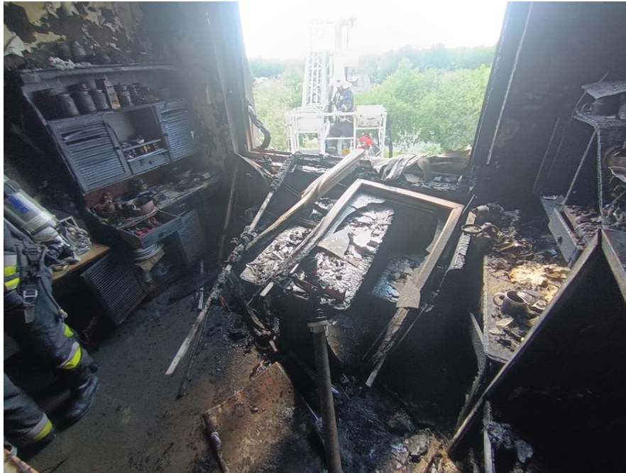
Figure 21/ MRSZ KMCS firefighters engaged in fire suppression operations in a mid-rise building.
