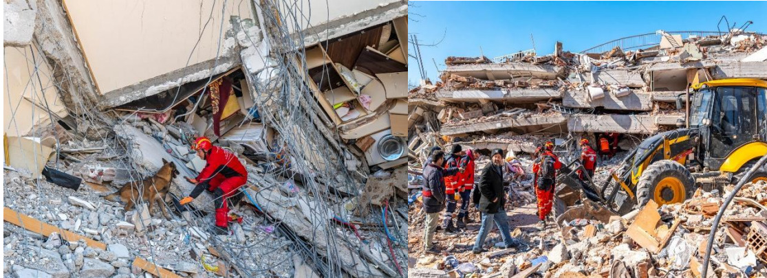
Figure 11: PUI team search and rescue on site in Türkiye, 2023. (2)
